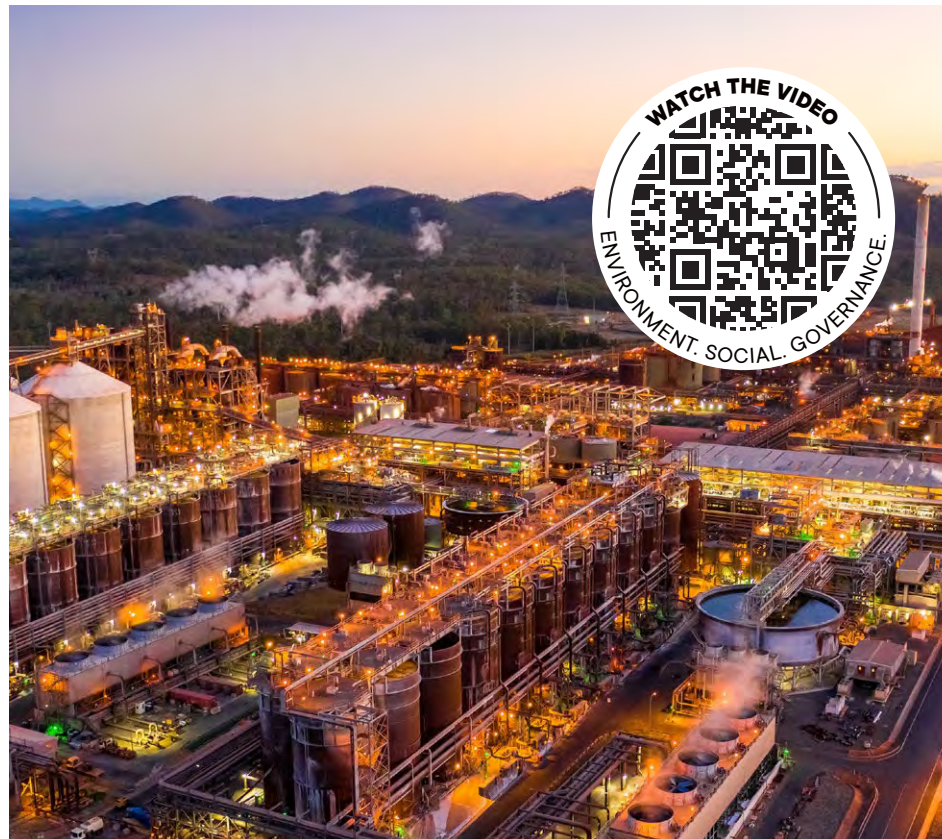
➔ Rio Tinto's Yarwun alumina refinery in Central Queensland.
